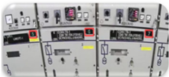
Panel no. verification through Optical character recognition (OCR)
