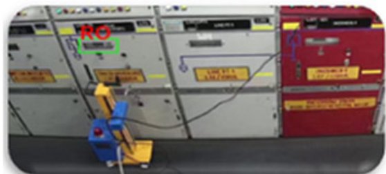
Autonomous Remote rack out detection
