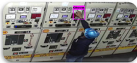
PPE noncompliance detected by system (Gloves)
